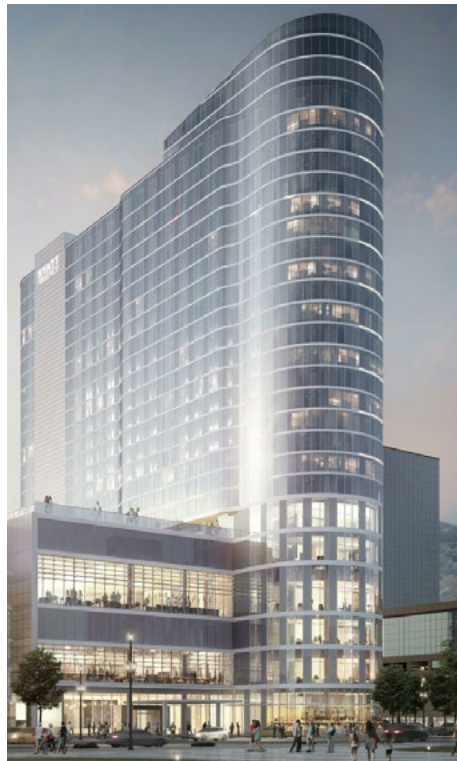
Salt Lake City Hotel : This 26- Story Tower includes: Two High Pressure Fire Pump Systems, Water Storage Tank, Standpipe systems, Dry, Pre Action and Wet systems.
